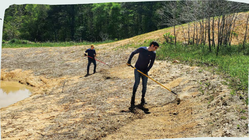
Benoit and Wyatt prepping the pond for erosion prevention
