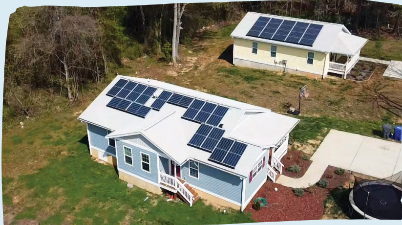
Two solar installs on Habitat Homes in Orange County, NC
